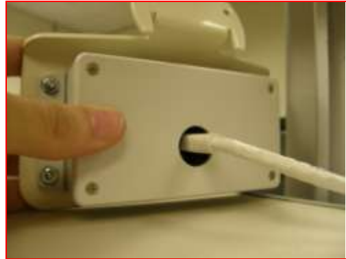
Figure 54. Cable plugged in
