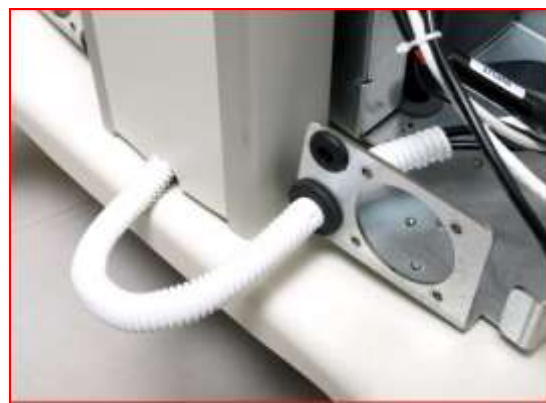
Figure 70. Installing wire loom
