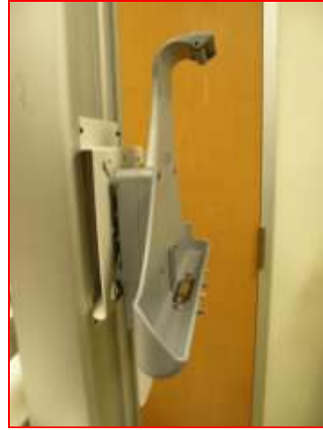
Figure 42. Placing 15" from top
