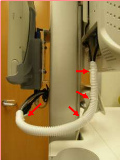
Figure 64. Installing wire loom
