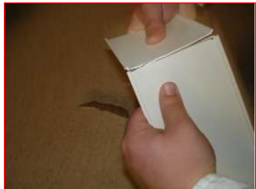
Figure 66. Snapping excess off
