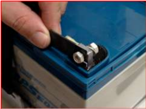
Figure 77. Placing Thermal Sensor
