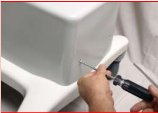
Figure 14. Removing Plastic Shroud
