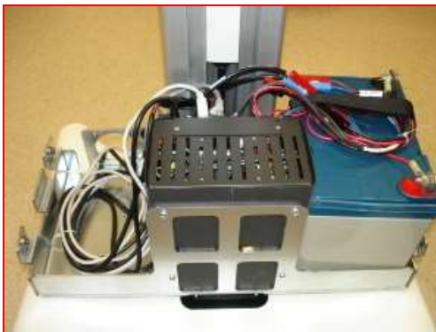
Figure 79. Securing Batteries and Cords
