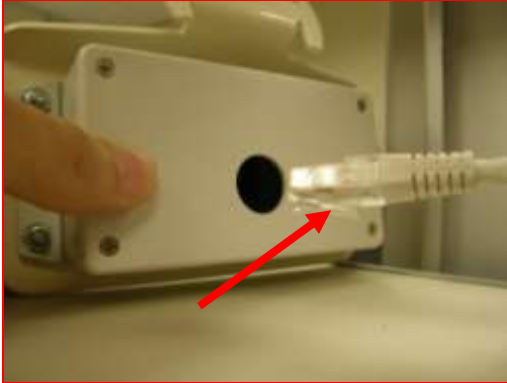
Figure 53. Plugging in cable
